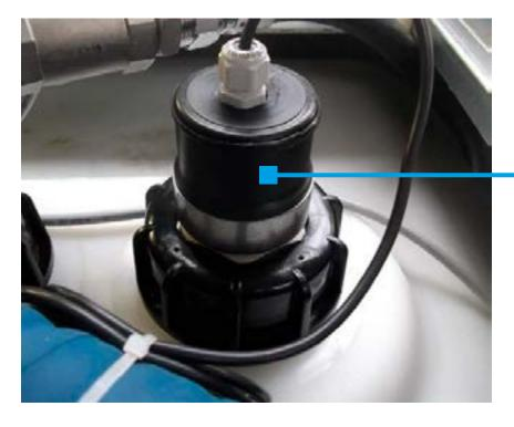
HOUSING FOR LEVEL MEASUREMENT PROBE
